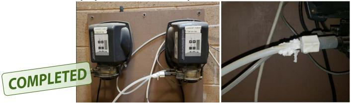
• The double containment tank is compromised by placing drain valves at bottom of tank through both walls. Leaks turned into build up on tank appurtenances. If the valve is breaks off, the tank contents will empty, defeating the double containment requirement.
