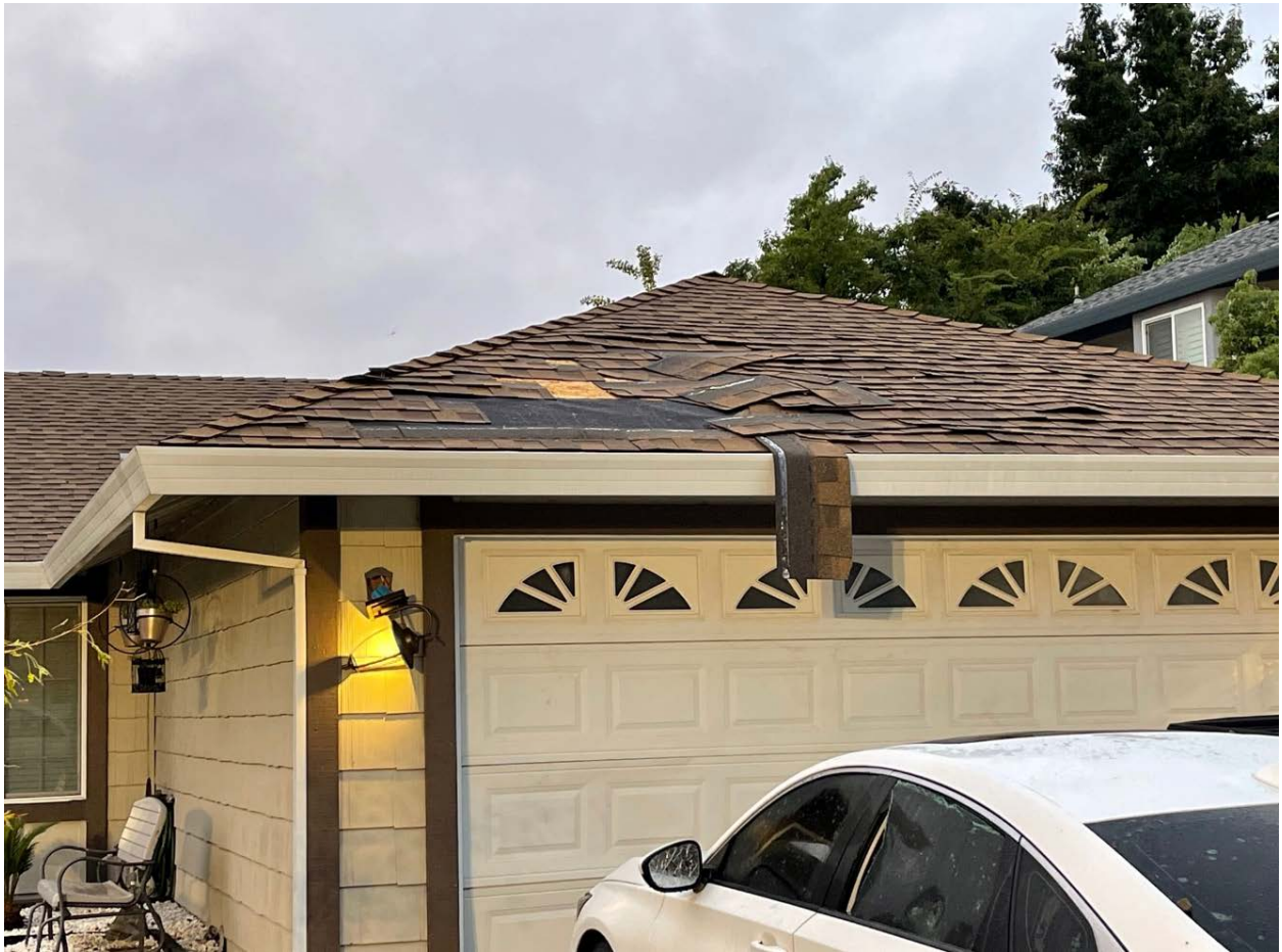
Damage caused by water main failure
