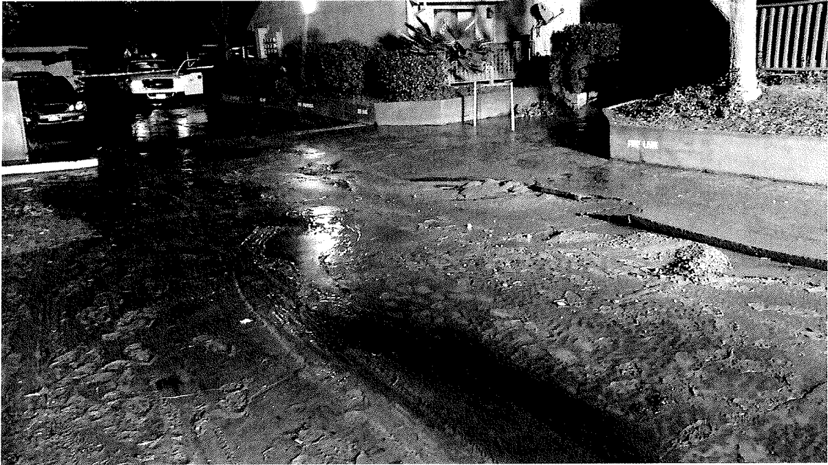
This photo of the entrance to the condominium complex shows the volume of dirt and gravel that was unearthed as a result of the water main failure.
