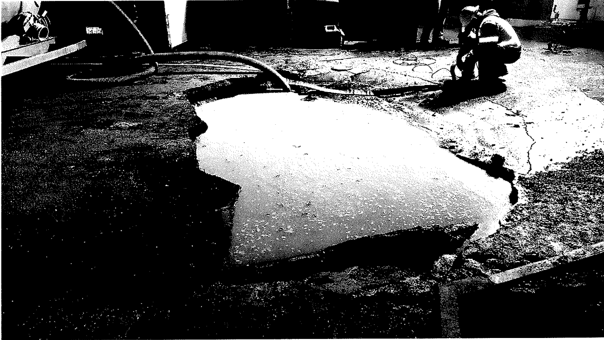
This photo illustrates the size of the initial cavity in the parking area excavated by the force of the water during the water main failure.
