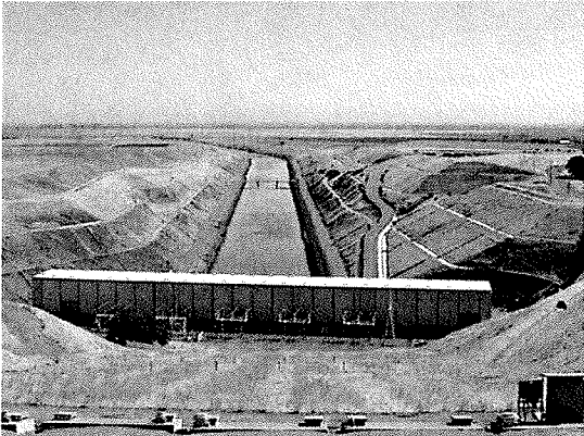
Banks Pumping Plant, part of the State Water Project Curtis Jerome Haynes / Courtesy
