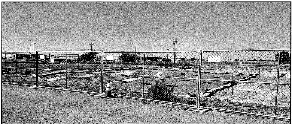
Initial excavation at CS067 was halted.
