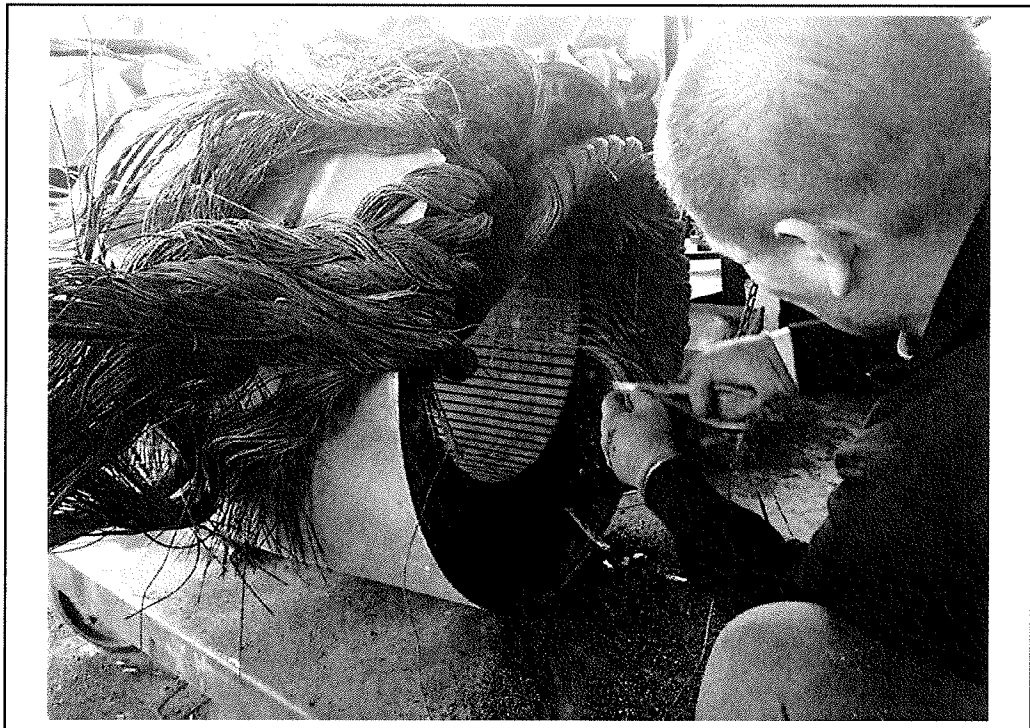
Figure 3 □ Well 56A Motor Winding Wire Removal
