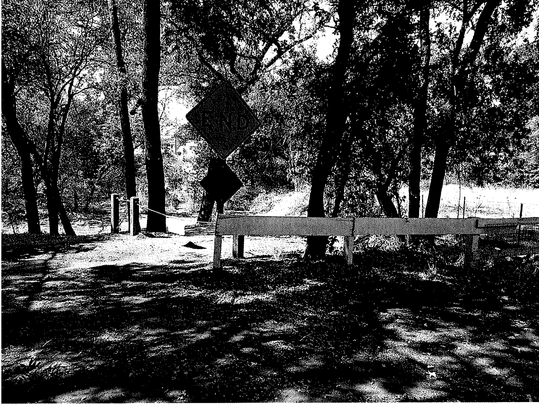
Above: Palm Avenue Right of Way cleared of garbage and 3 wooden bollards with cables installed.
