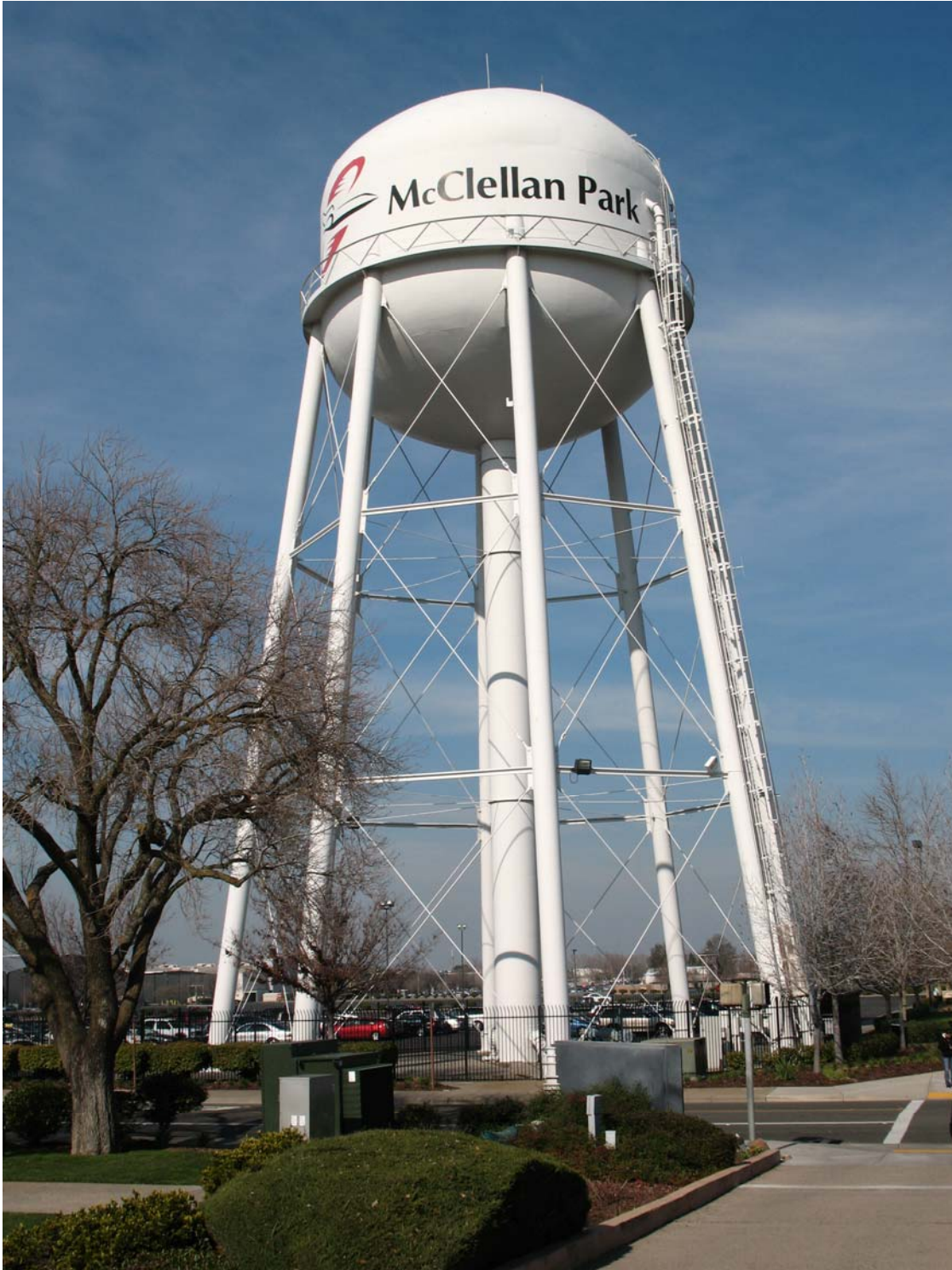
McClellan Business Park Elevated Tank #216 (0.5 MG)
