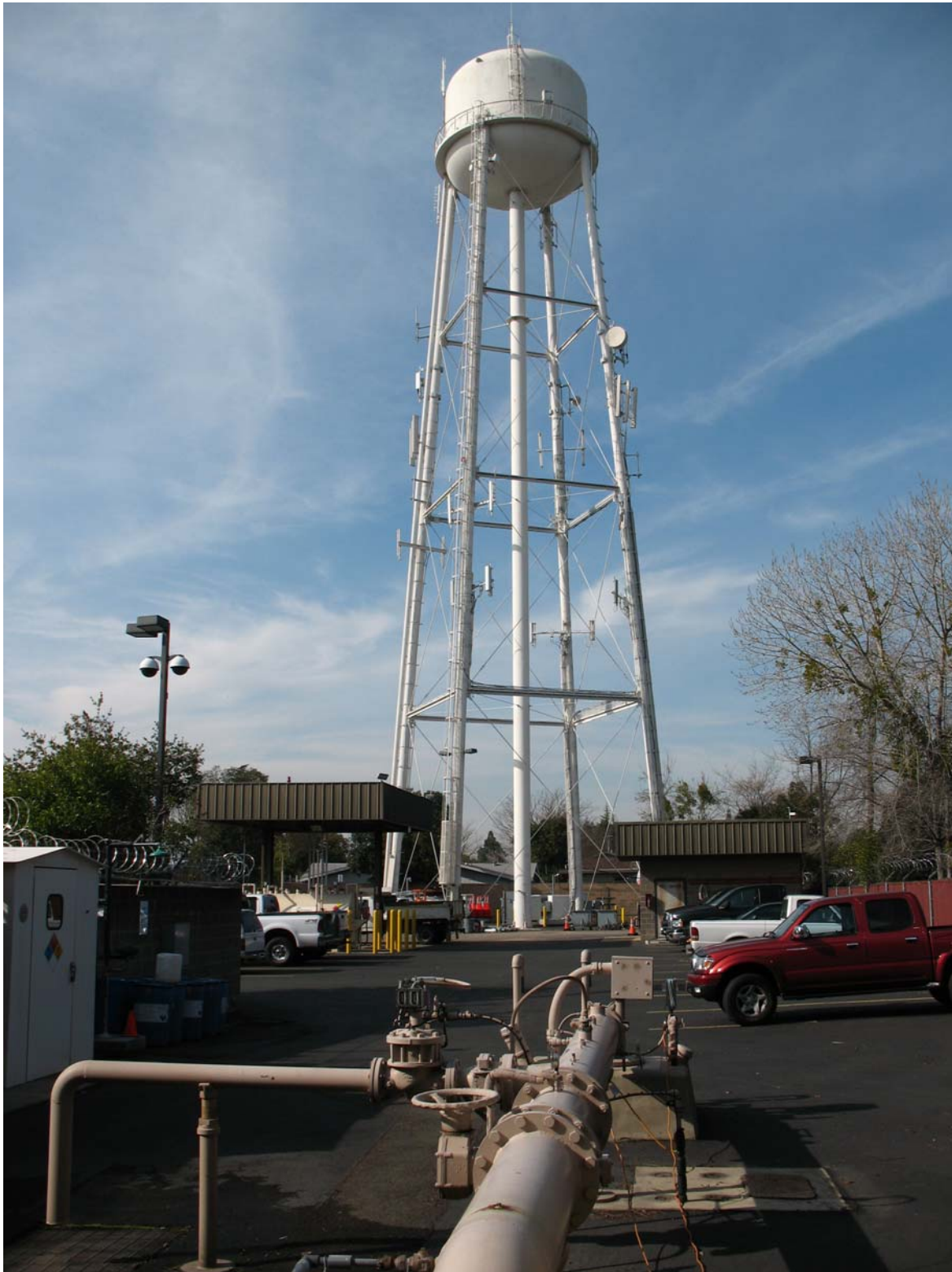
Walnut Yard Elevated Tank (0.125 MG)
