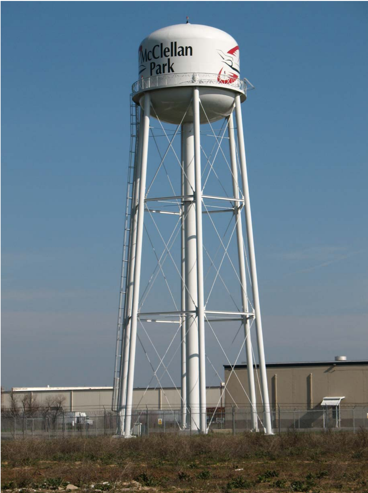
McClellan Business Park Elevated Tank #769 (0.15 MG)
