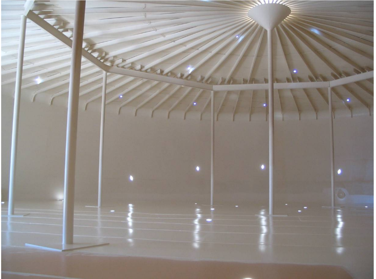
Enterprise/Northrop Reservoir (5 MG) – Photo of Tank Interior After Construction in 2006
