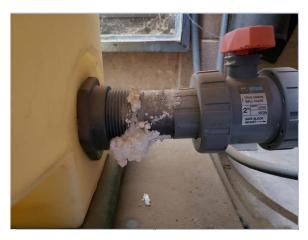
• Sodium Hypochlorite Tank will drain if ball valve opens, fails, or breaks off.
