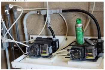
• Chemical pumps have leaks and build up. Rags are used to absorb chemical drips.
