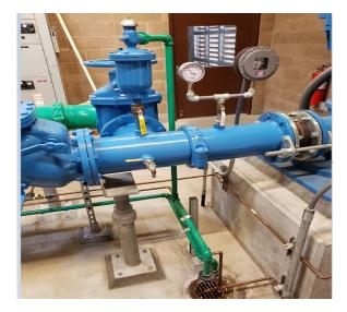
• Raw water sample ports are not threaded, but they are barbed. Required by DDW based upon *Chapter 16 – California Waterworks Standards - Article3 - Water Sources §64560*
