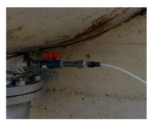
• The pump base Air Release Valve (ARV) discharge does not meet the minimum required 36" from ground surface. Reference: Water Well Standards (Bulletins 74-81 & 74-91) – Section 10, Surface Construction Features.
