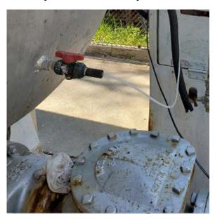
• There are no identifiers of what is contained within this locked container. This is where the liquid sodium hypochlorite is stored.
