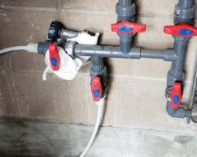
• Chemical degas pump discharges into an open bucket.
