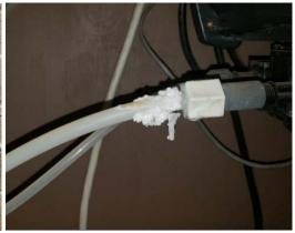
• The double containment tank is compromised by placing drain valves at bottom of tank through both walls. Leaks turned into build up on tank appurtenances. If the valve is breaks off, the tank contents will empty, defeating the double containment requirement.
