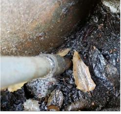
• Pump base seal is separating. When the well turns off, contaminants could potentially be sucked into the aquifer.
