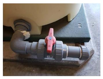
• There is no double containment on pressurized tubing and there are leaks where the tubing connects to the PVC piping. Lubricant spray was left sitting on top of chemical dosing pump.
