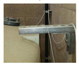
• Instead of double containment, tubs and lids that are placed to catch drips.
