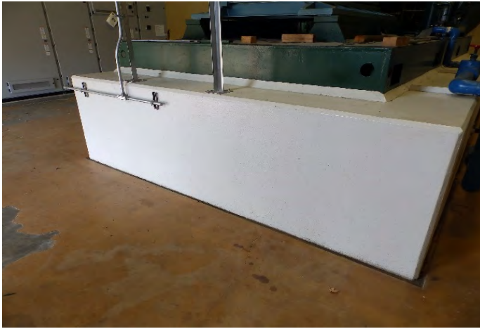
Structural Asset in Excellent Condition: Score = 1
